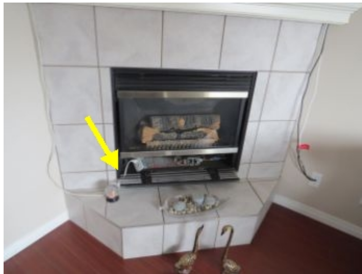
Dangerous to use extension cord at this location.
