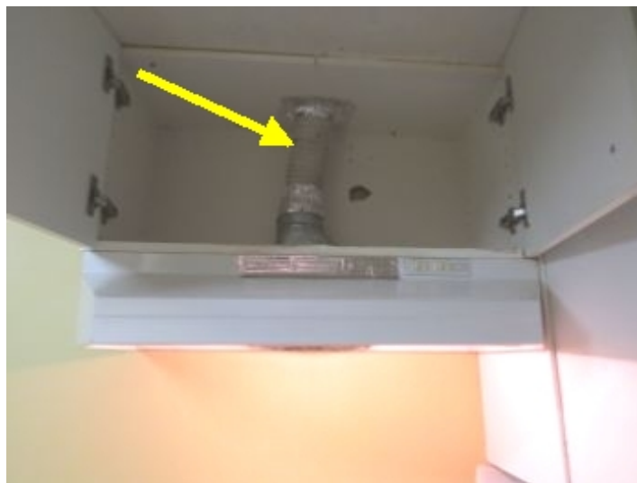
Vent must be metal &amp; correct size
