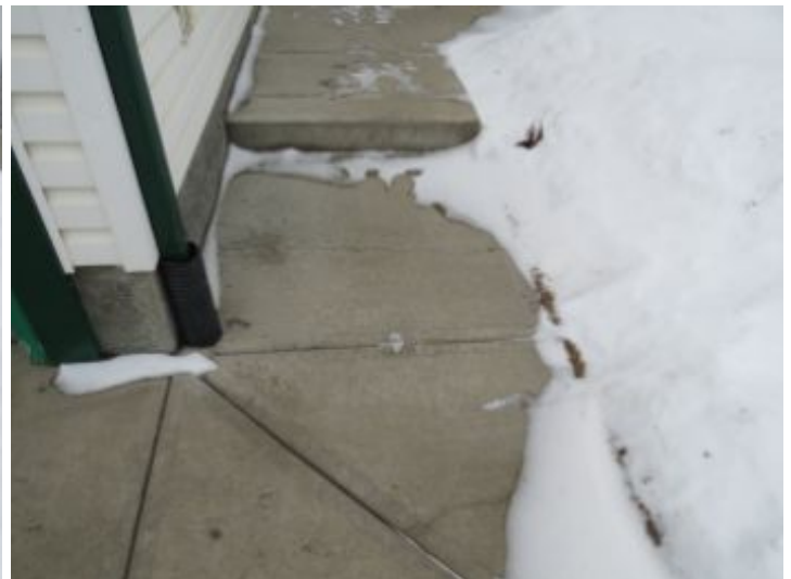
Concrete cracks
