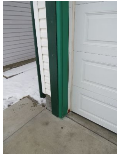
Repair/replace weather stripping
