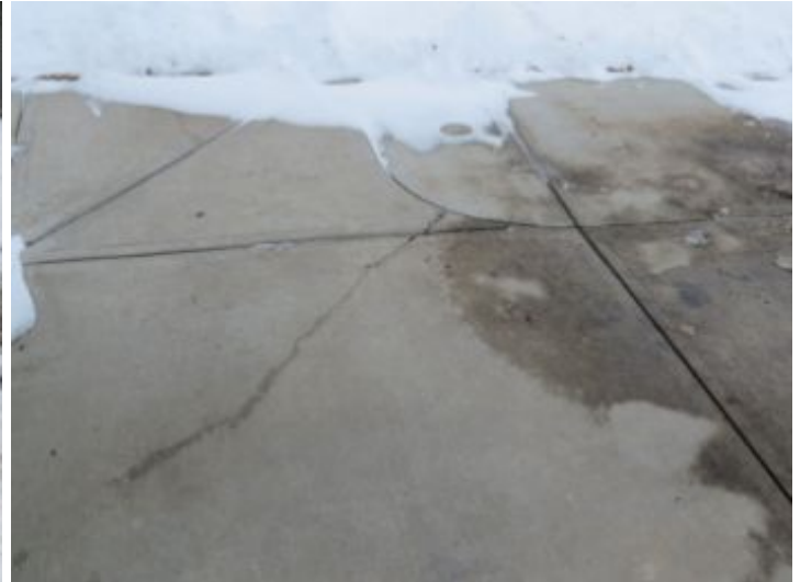
Concrete cracks
