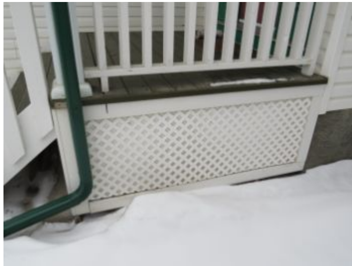
No access to the underside
